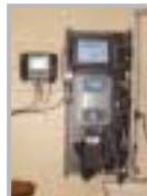
The Hach Water Distribution Monitoring Panel (WDMPsc) is a compact panel fitted with four analyzers to monitor free or total chlorine, turbidity, pH, conductivity, temperature and sample pressure. NWWA's SCADA system collects data continuously from its six monitoring panels, allowing for comprehensive water quality network surveillance at all times.
